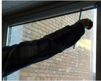
6: Spray the film surface with the water and soap solution. Use the recommended squeegee, and push it across the film using both hands at a 20-30° downward angle, to remove any remaining water under the film.
